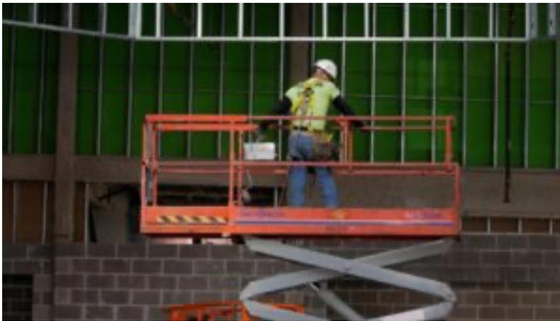
Group classification is determined by whether the lift stays within the tipping lines or moves beyond the tipping lines. “Group A” MEWPs move vertically but stay within the chassis or tipping lines. Scissor lifts are an example of this group. “Group B” MEWPs can move beyond the machine’s chassis or tipping lines (wheels or outriggers). Group B generally refers to boom lifts.
