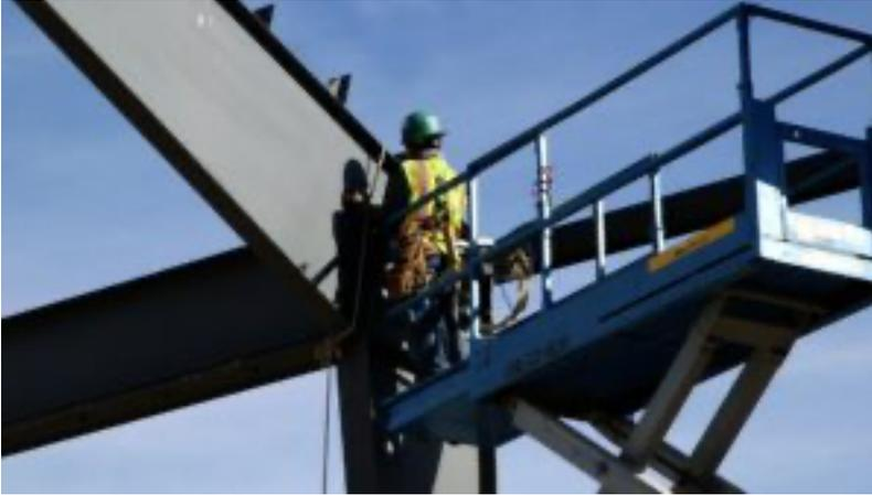
entrance gates, taller platform railings, and sustained involuntary operation controls. Operators must be familiarized with the MEWPs being used and trained on the new safety features prior to operating. Existing equipment is not required to be retrofitted to meet the new design requirements. Therefore, it is important for all employees to know the differences between the company's various MEWPs and are properly trained on both as needed.
